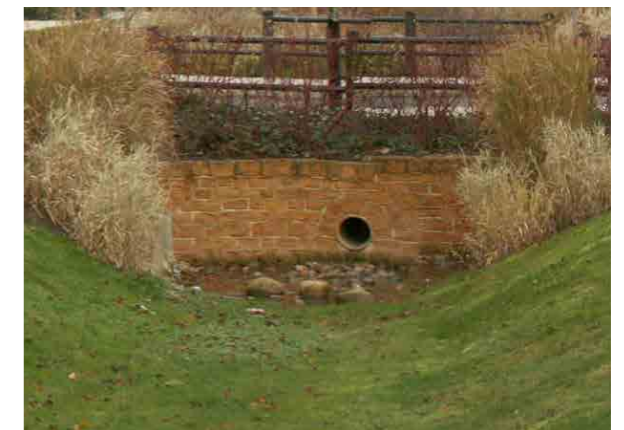
Stone head walls within landscaped areas.
