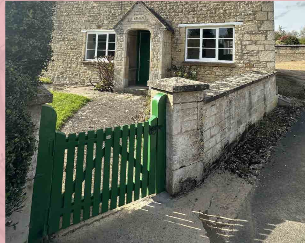
Reconstituted stone rubble wall with capping will be used to enclose front areas of hot buildings as seen in Great Oakley Village.
