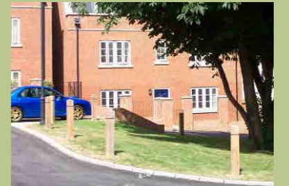
Timber posts to edge of green space.
