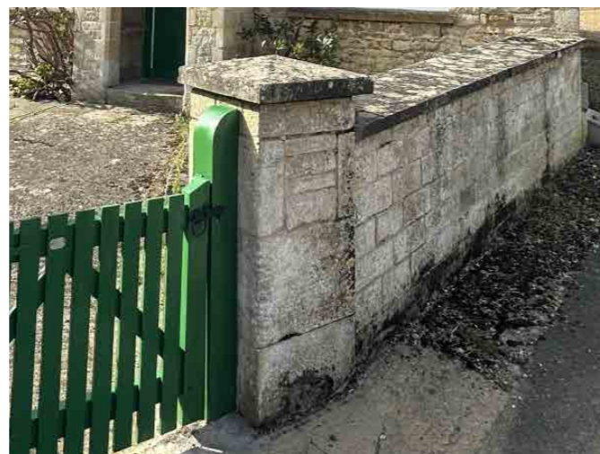
Natural low stone wall fronting hot buildings.
