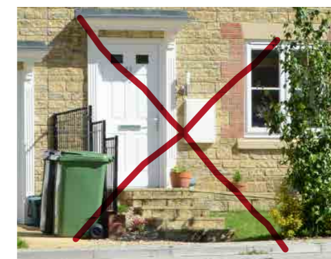
Meter boxes on the front of a building should be avoided where possible.
