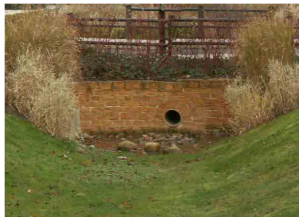
Stone head walls within landscaped areas
