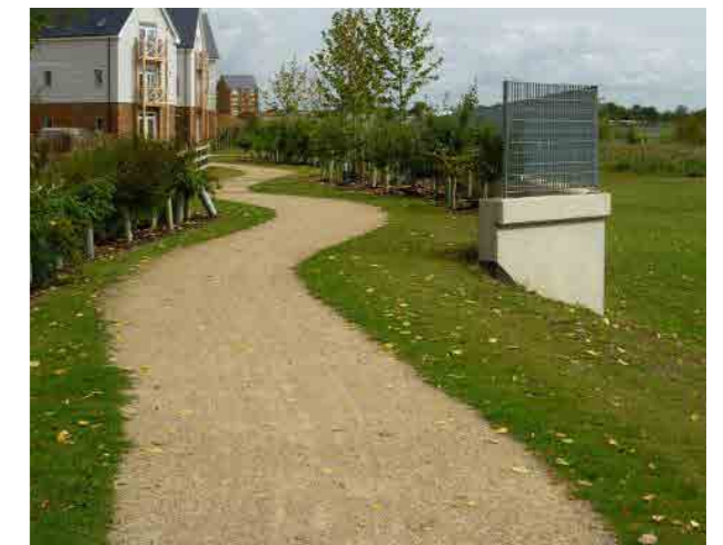
Self binding stone surface.
