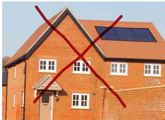
PV raised panel on a bright red tile roof.
