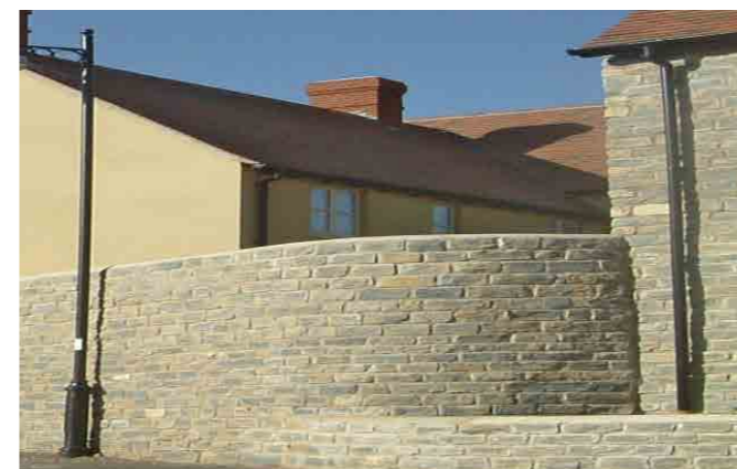
Example of side wall material matching the house.
