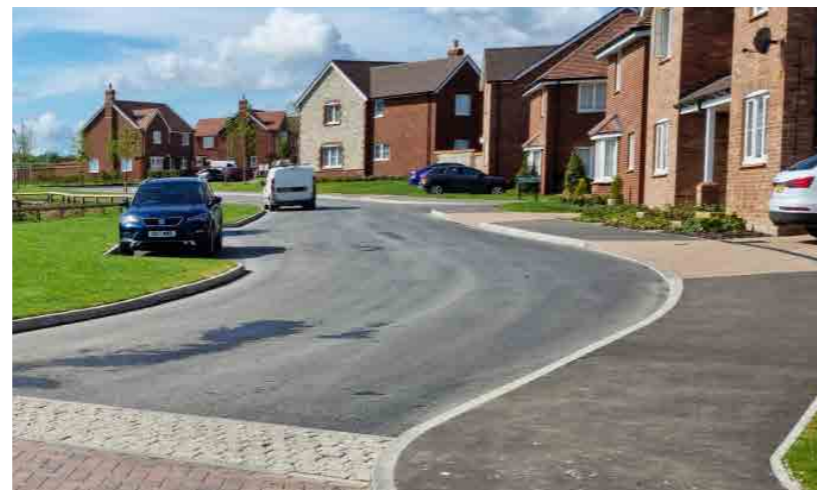
Bitumen macadam to road and pavements.
